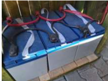
Figure 9. The battery group of the solar-based automatic pet feeder and water dispenser in use
