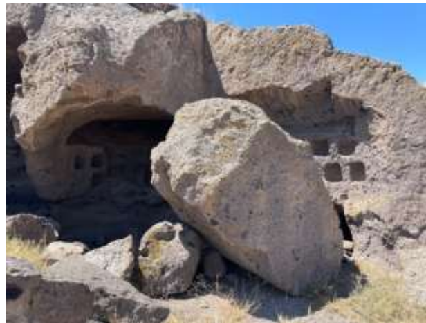
Figure 3. Block breaks caused by cracks
