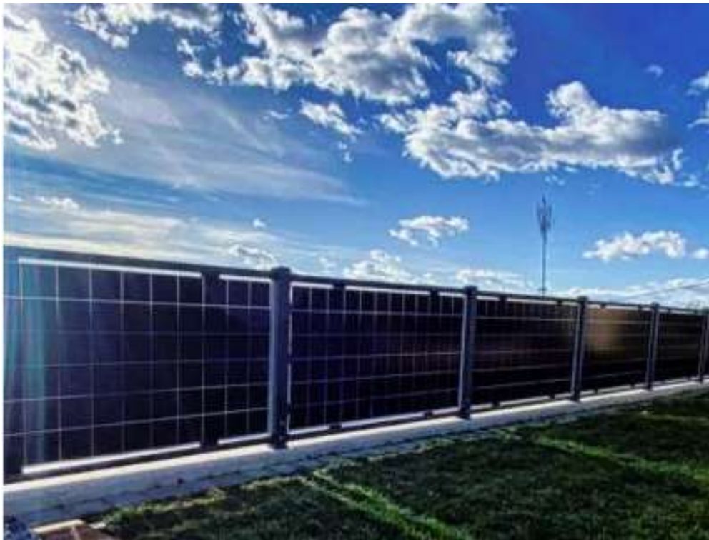
Figure 2. Application model of a fence made of solar panels ( www.next2sun.com ).
