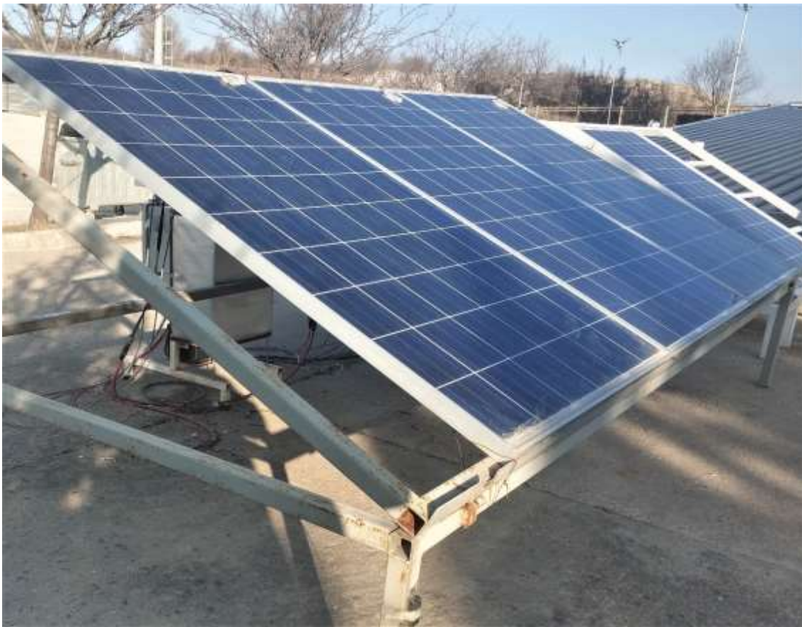
Figure 2. Photovoltaic Panel Installation
