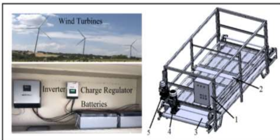
Figure 1. Wind Turbine and vermicompost production facility 1. Control Panel 2. Double bladed manure harvesting knife 3. Conveyor band 4. Electric motor operating the knife 5. Electric motor operating the conveyor band
