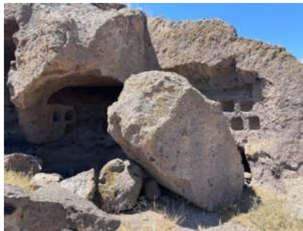
Figure 3. Block breaks caused by cracks
