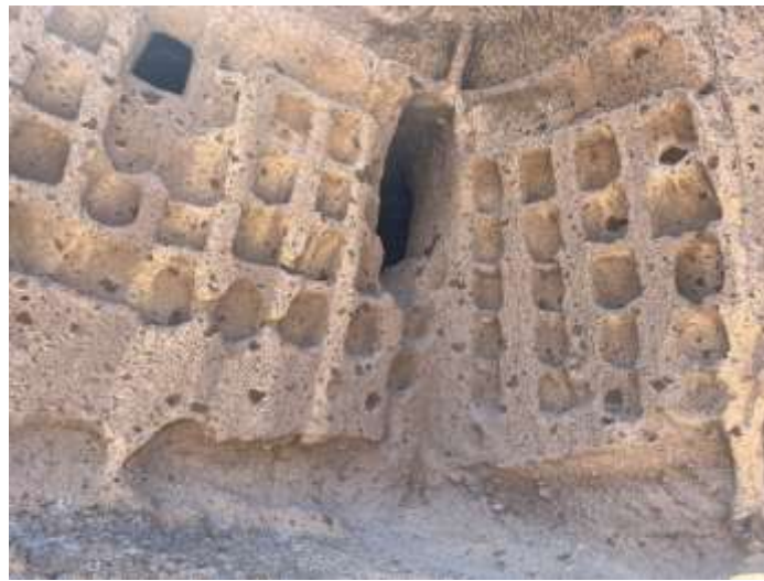
Figure 1. Differential erosion and missing part type deteriorations observed in the Şahmelik Tuff Rock Monument
