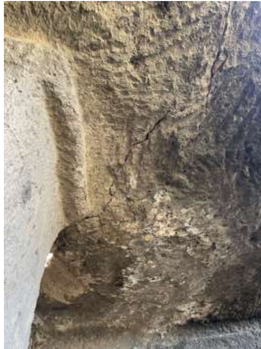
Figure 2. Crack type deteriorations observed in the monument
