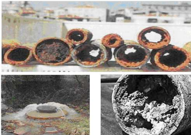
Picture 1. Destruction of oils in pipes
