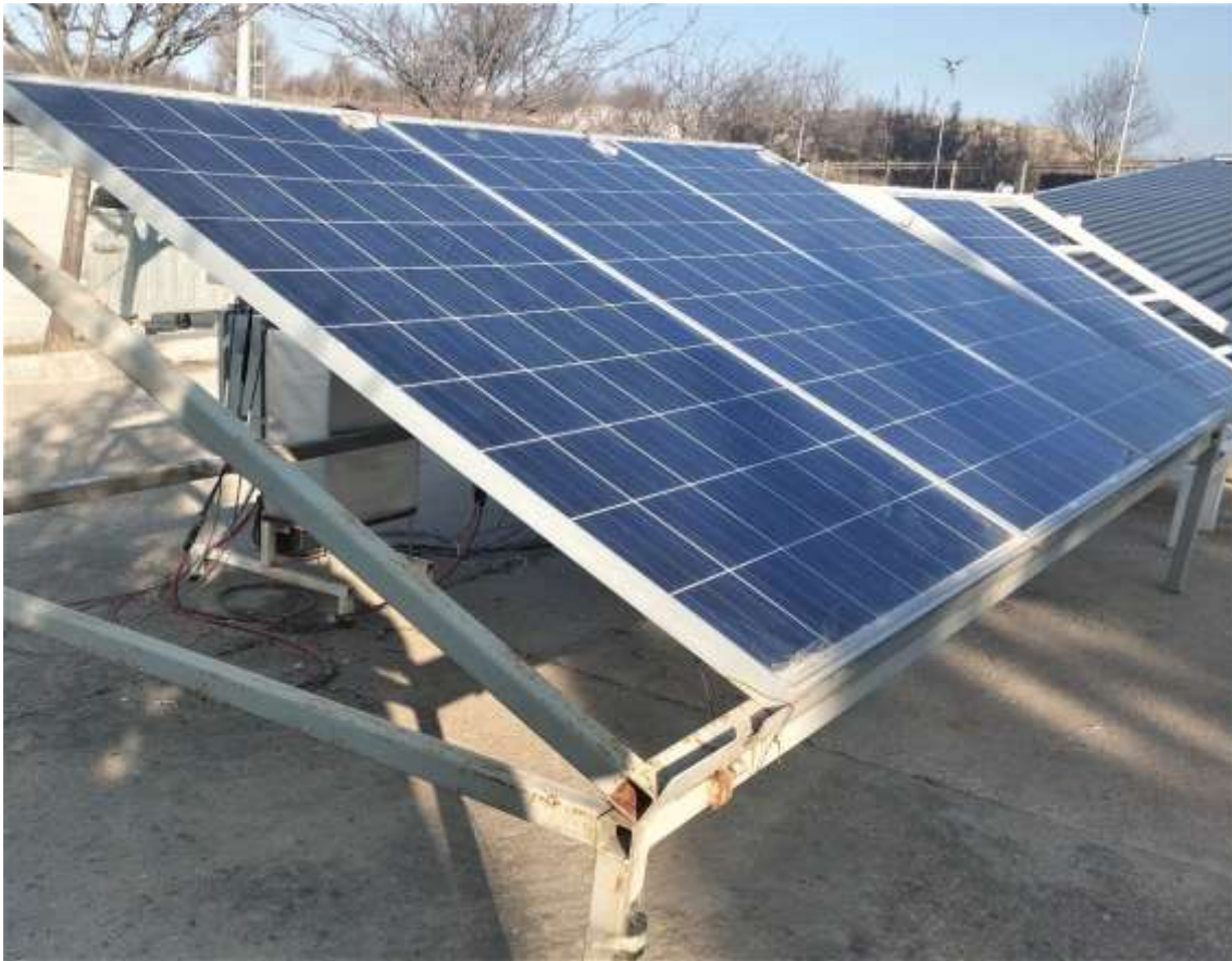
Figure 2. Photovoltaic Panel Installation
